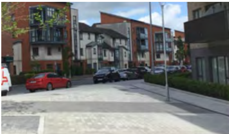
Exposed aggregate panels with natural stone banding matching historic public realm finishes at Phibsborough Centre ACA.
